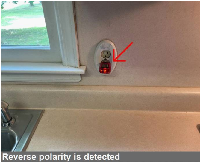
Reverse polarity is detected
