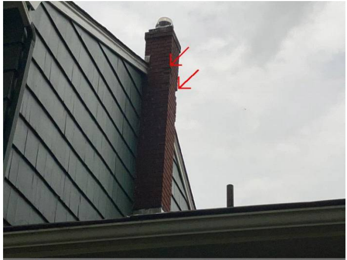
spalling (cracking) of the bricks
