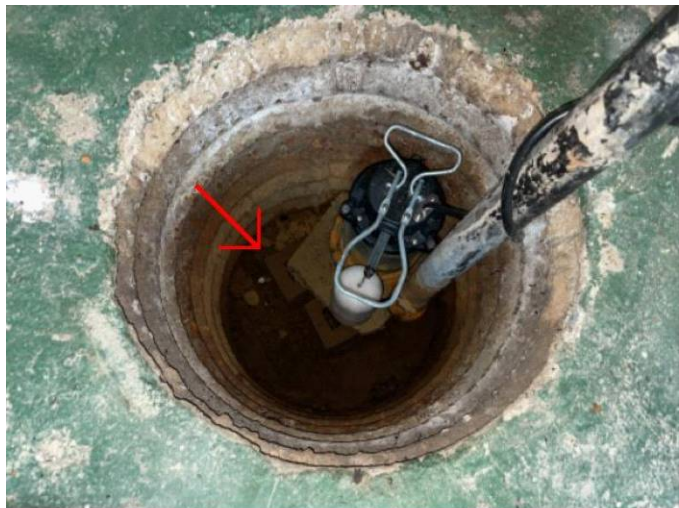
indications of water leakage | sump pit
