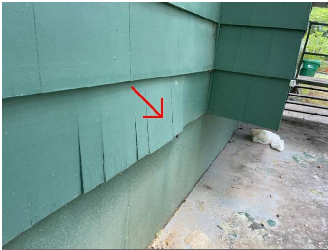
loose fastened exterior siding
