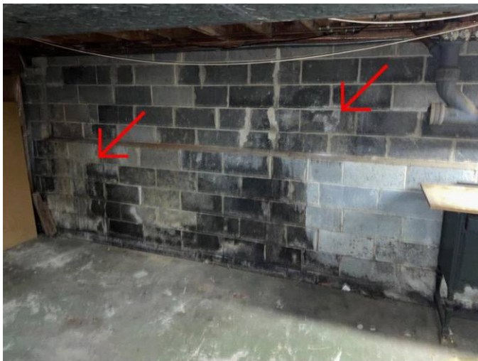
indications of water leakage
