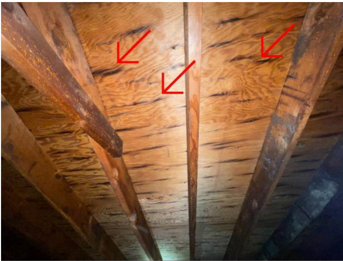
suspected mold forming
