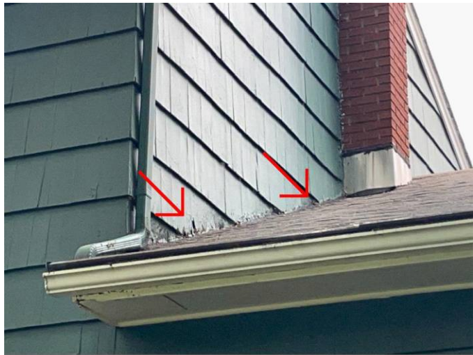
rotted exterior siding
