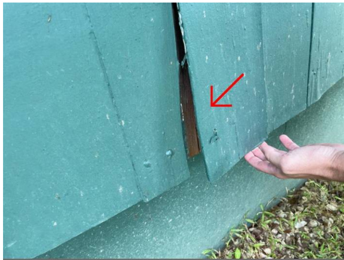
inadequately fastened exterior siding
