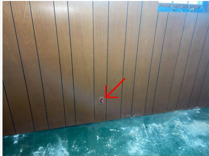
Reverse polarity is detected
