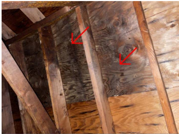
suspected mold forming
