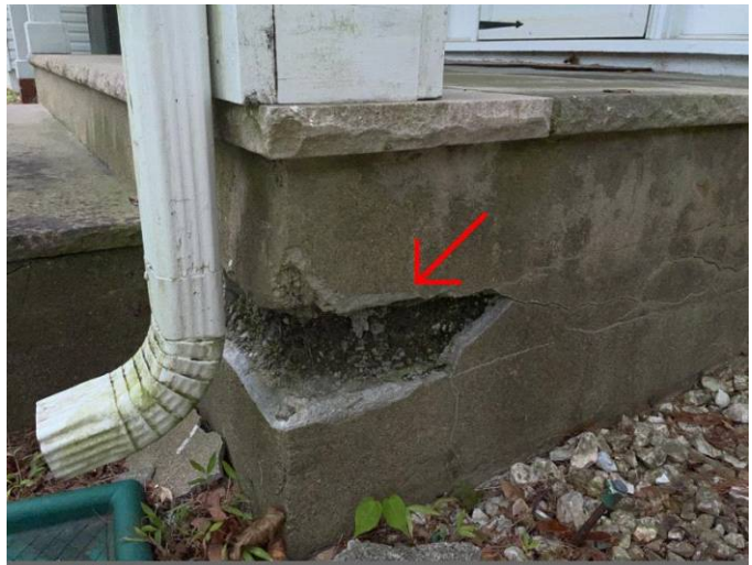
cracking masonry
