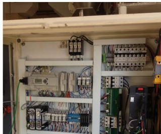
After - The brand-new Allen Bradley PLC based control panel with Servo drives is installed.
