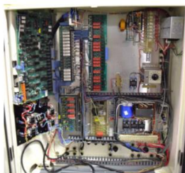
Before - The old Hayssen main control panels removed. Input/Output wiring is disconnected
