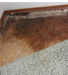
Leak Under The Floor
