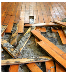
Leak Under The Floor
