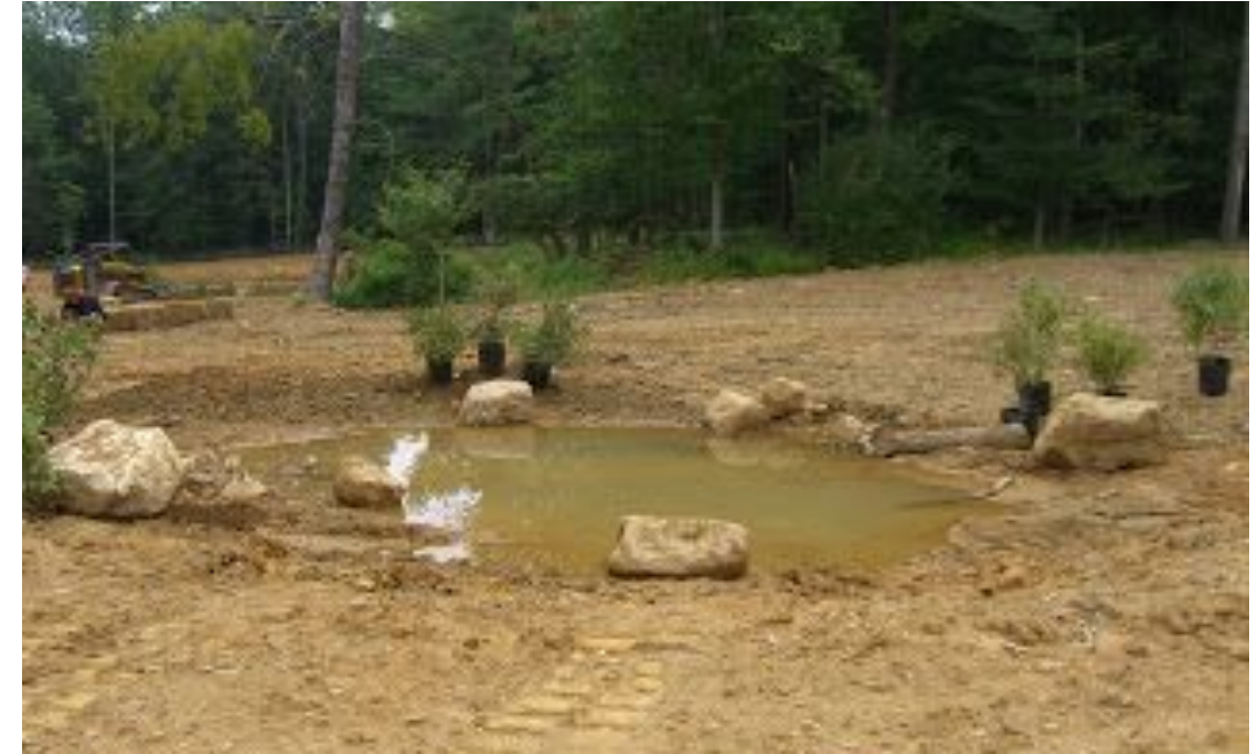
A poorly drained site being prepared for a native plant installation.
