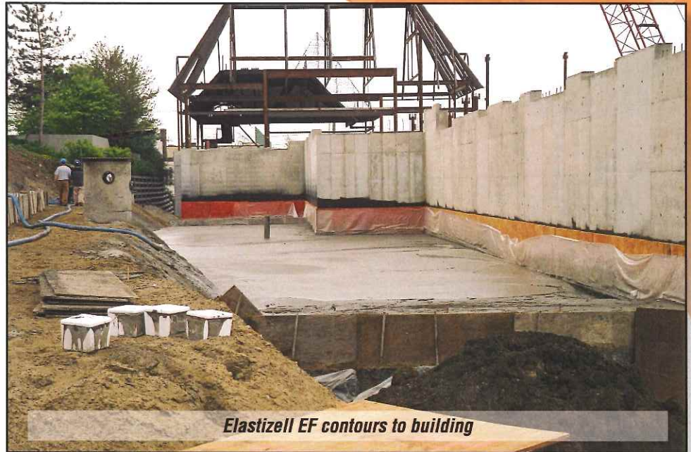
Elastizell EF basement backfill placement
