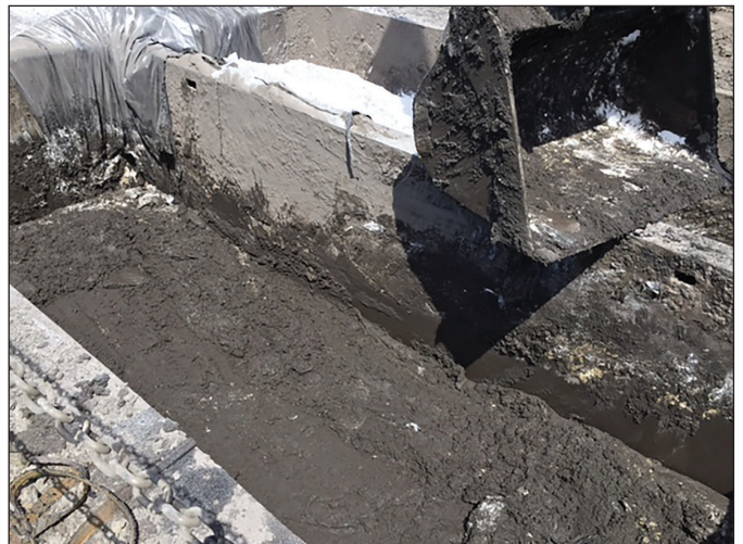
Using perlite in a large-scale liquid waste solidification process.
