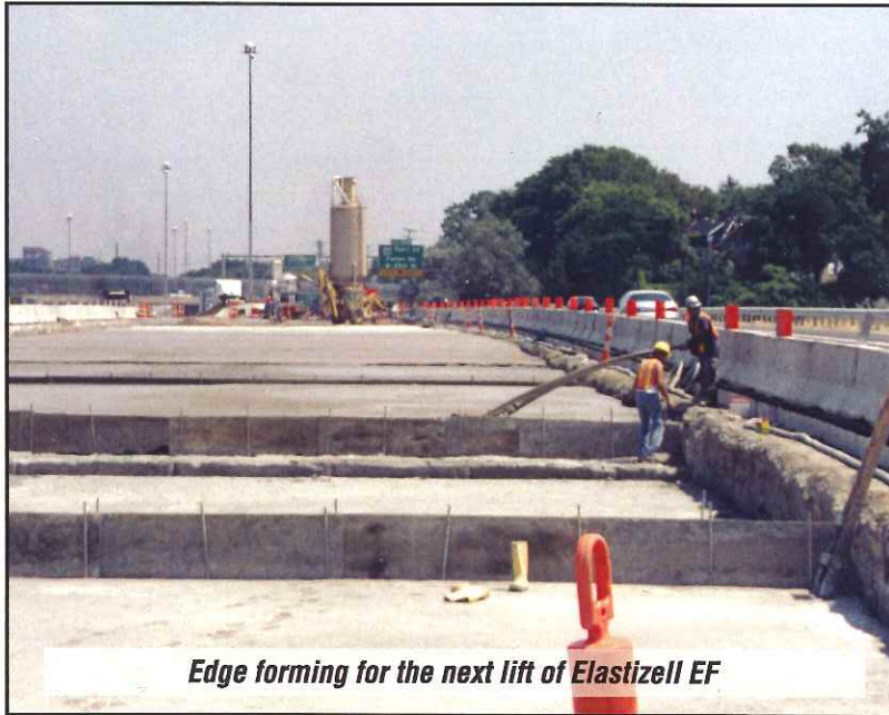
Self leveling and compaction free placement of Elastizell EF
