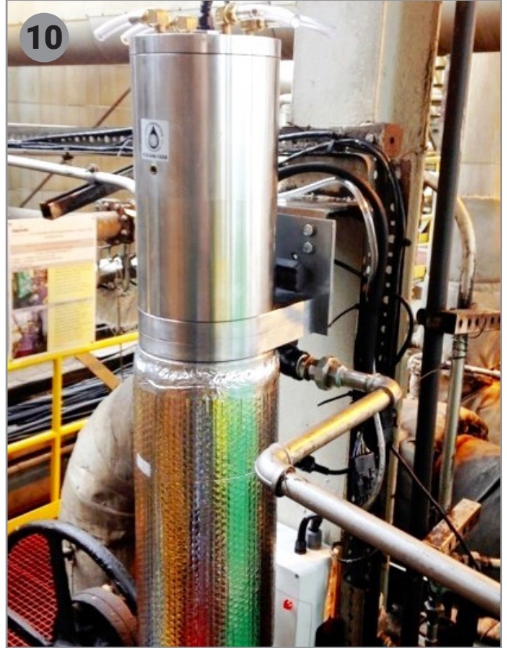
10. The Conserver® Oil Purification System cleans and dries oil and hydraulic fluids – extending drainage periods dramatically and reducing equipment and engine wear. In this photo a single H14 Conserver® Unit is mounted near a 100-gallon reservoir.
