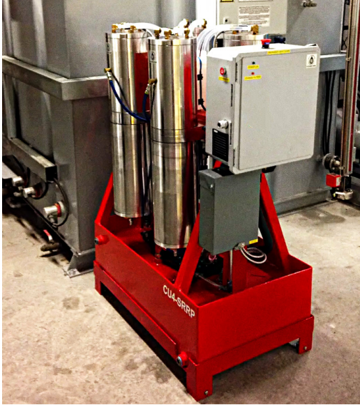
Four HI4 Generation 5 Conserver® units mounted on a stationary skid installed near a 900-gallon reservoir at a paper mill. The system control box supplies the necessary logic and controls to ensure the unit performs properly.
