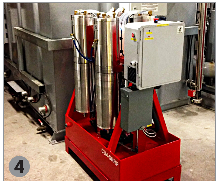
4. Four HI4 Conserver® units mounted on a custom stationary skid. The system is installed near a large reservoir at a paper mill.
