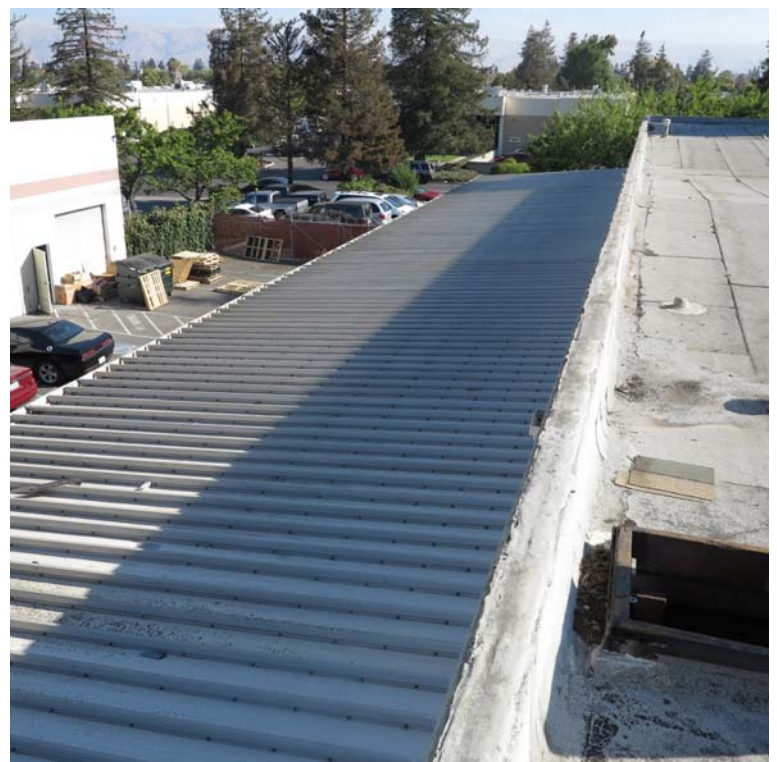
Metal roof at the north end of the bldg.
