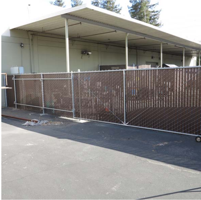
Rolling gate at 3310.
