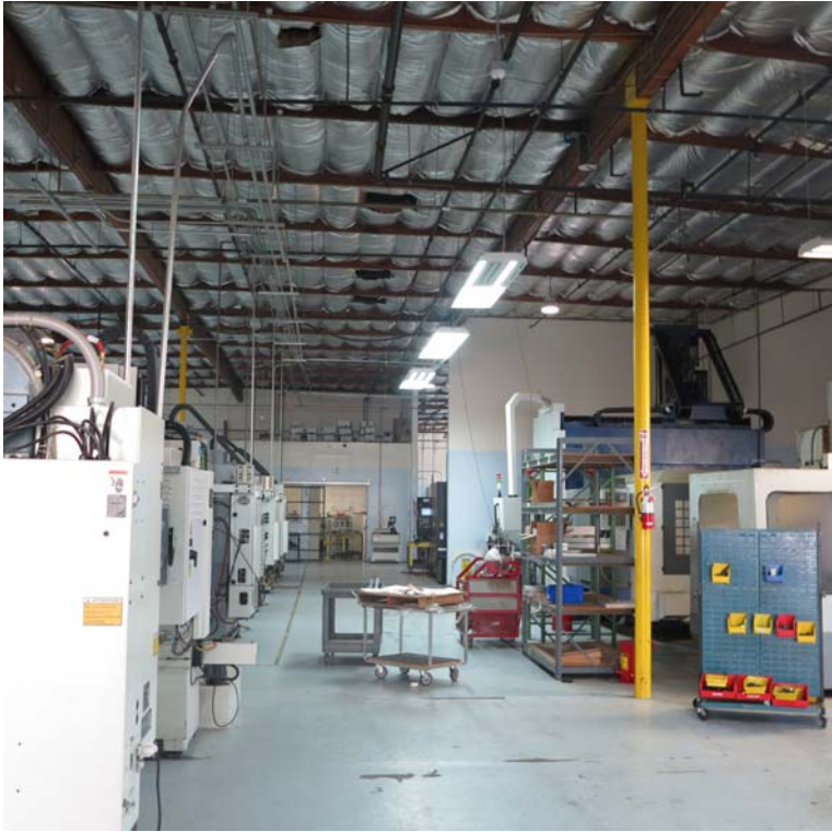
View showing lines of structural columns bearing the roof
