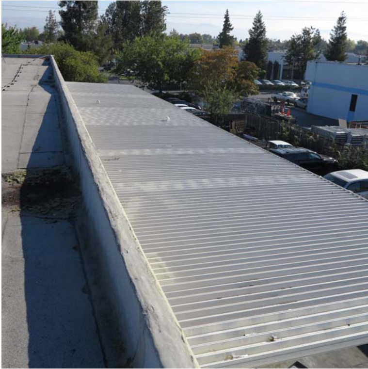
Metal roof at the south side of the bldg.
