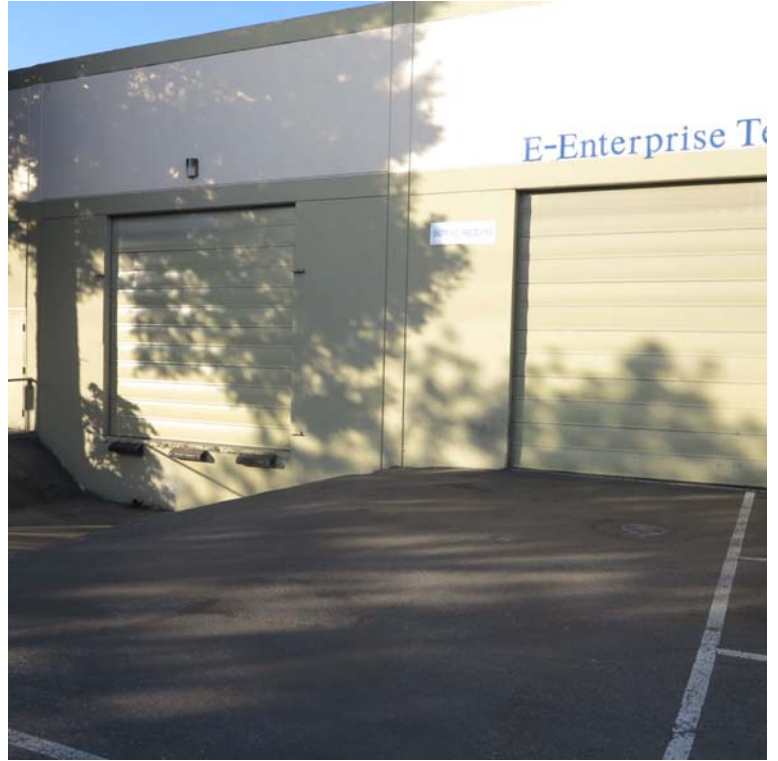
Dock high and grade level doors on the northeast end of the bldg.
