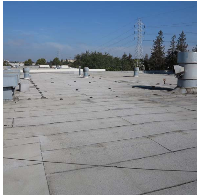
View of the roof looking north
