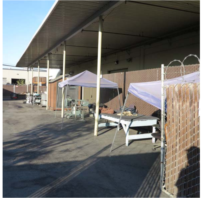
Overhang and yard area at south end of the bldg. (3310)
