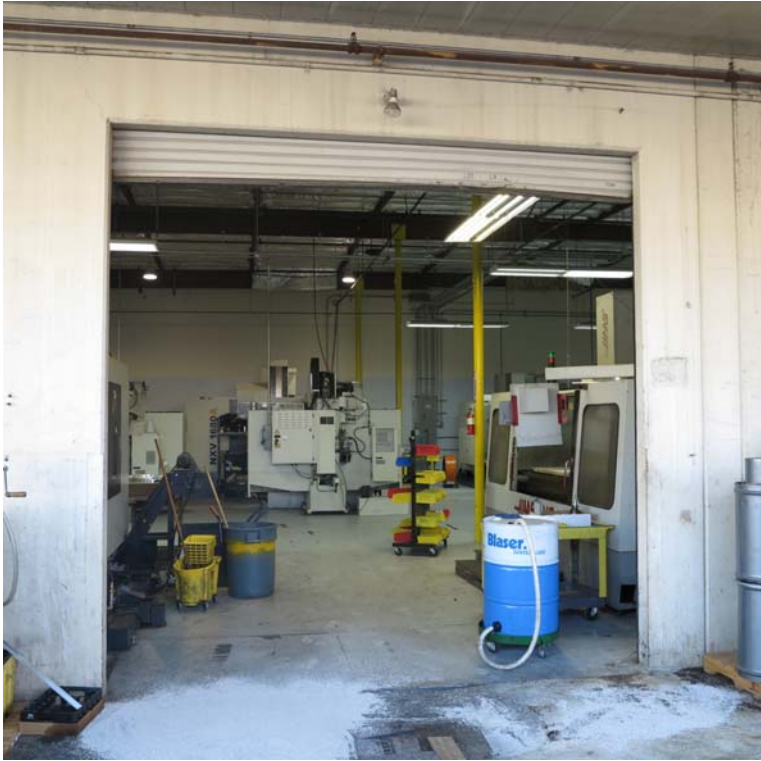
Grade level door at 3314, north end, typical , all appear to work. Chain hoist
