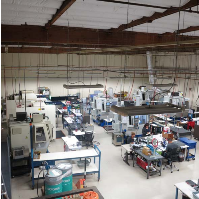
Mfg floor in 3310, Building roof insulated through out
