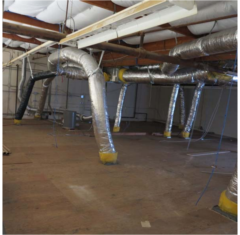
Above the hard lid ceiling in 3310
