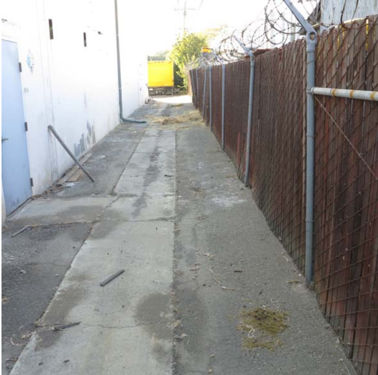
Concrete swale to carry away water at the west portion of 3310
