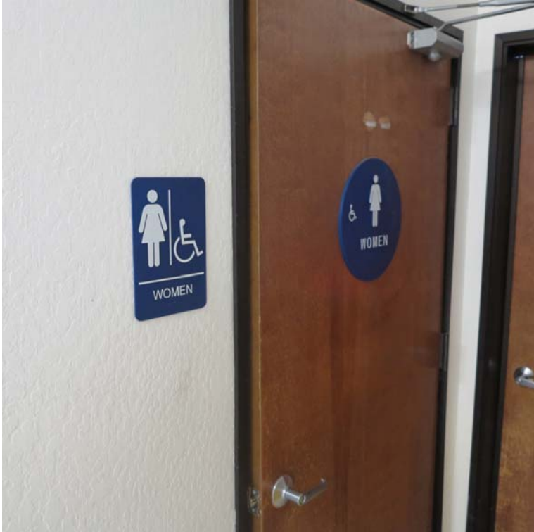
Example of correct signage
