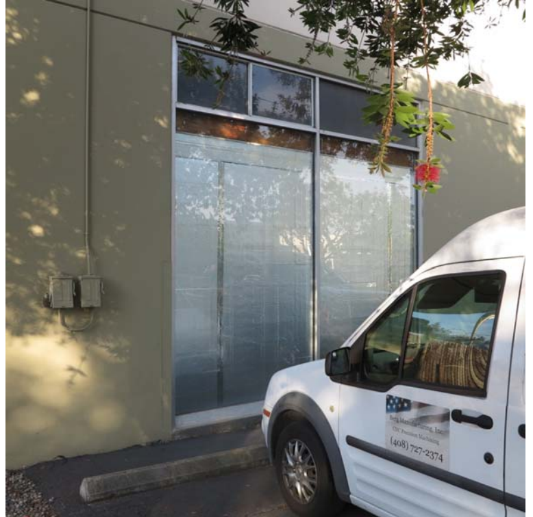
Grade level door filled in with glass at 3310
