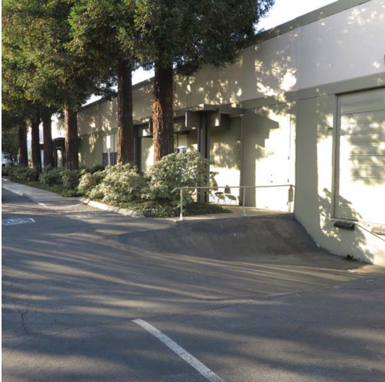
East (front) side of building
