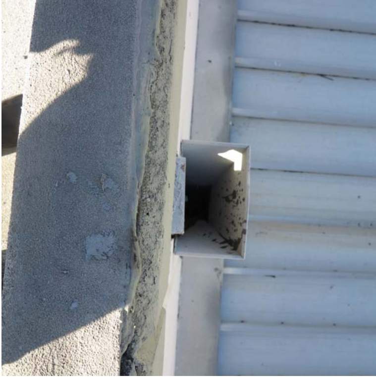
Through wall scupper
