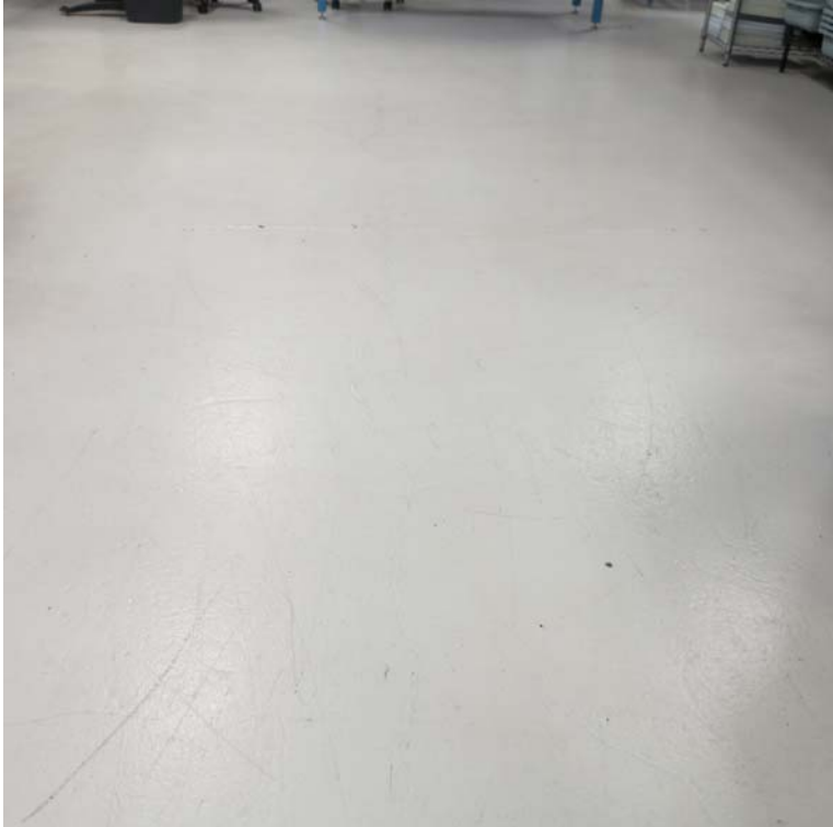
Painted concrete floor in 3310
