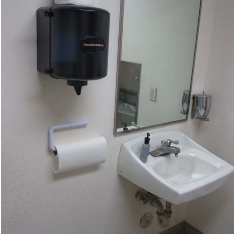
Shows HC compliant paper towel dispenser
