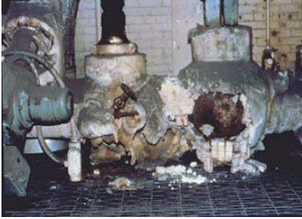
Valves insulated with asbestos
