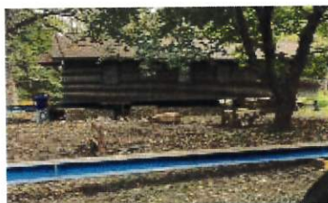
Moving Cabin 9 to make room for a NEW Cabin!
