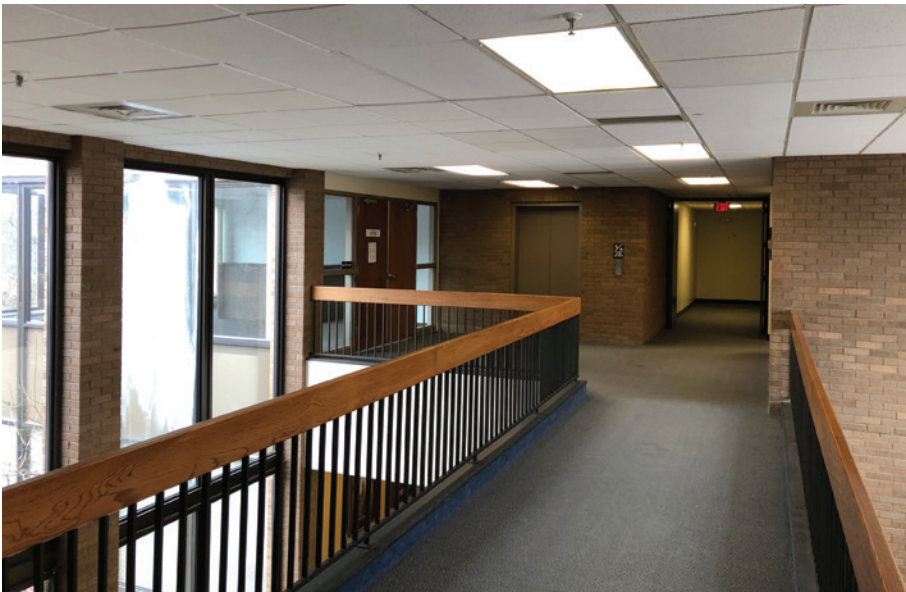
Before photo provided by Dimit Architects
