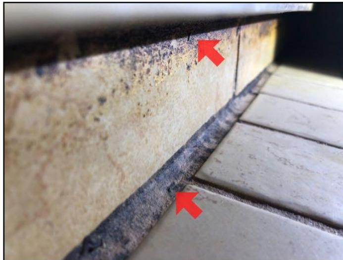
*Grout stained with mold*
