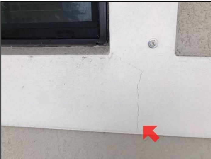
Exterior wall has minor/typical shrinkage...
