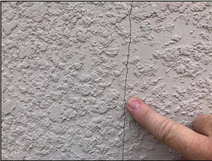
Exterior wall has minor/typical shrinkage...
