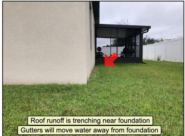
*Runoff eroding soil*
