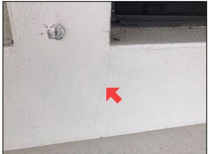
Exterior wall has minor/typical shrinkage...
