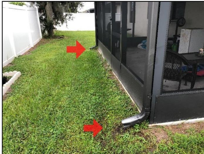
*Splashblock missing at gutter discharge...*
