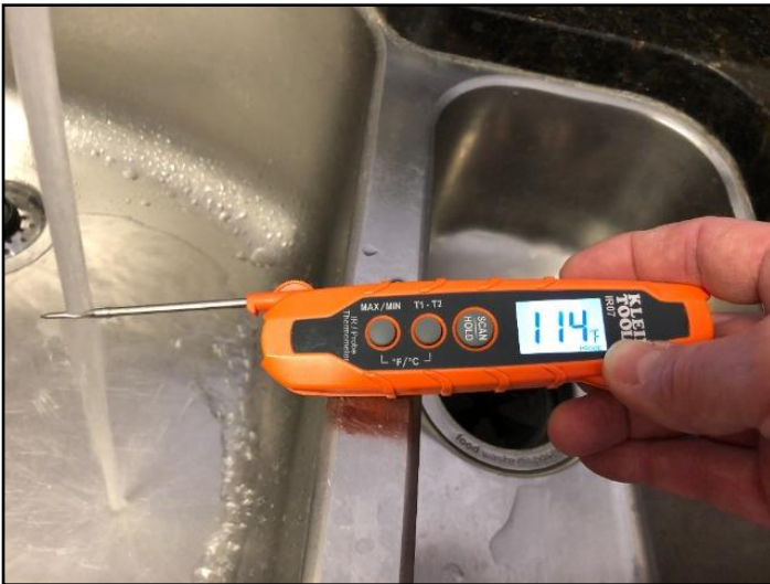
Water temp at kitchen sink
