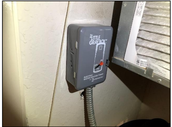
Water heater timer
