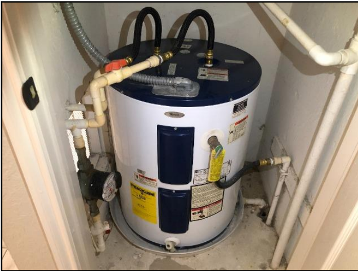
Conventional water heater
