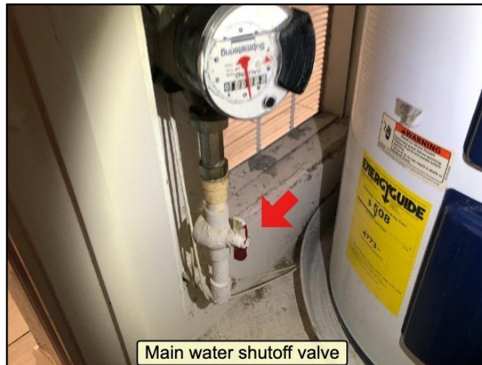
Main water shutoff valve
