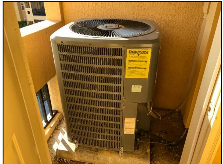
A/C Condenser on patio
