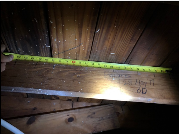
Roof Sheathing Nail Spacing Nail spacing is minimum of one per board
