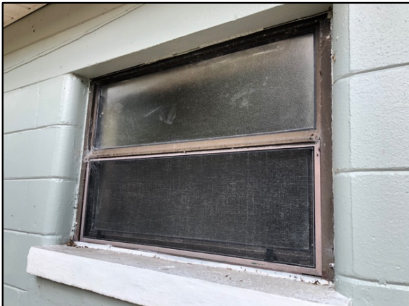
Windows are single pane and not impact rated
