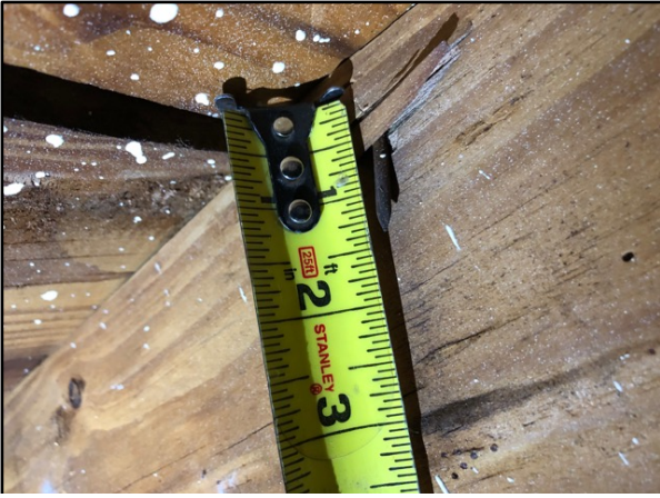
Roof Sheathing Nail Size Nail Size 6D
