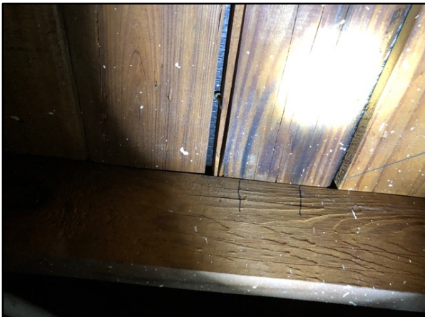
Roof Plywood Thickness Dimensional Lumber Thickness 1/2"
