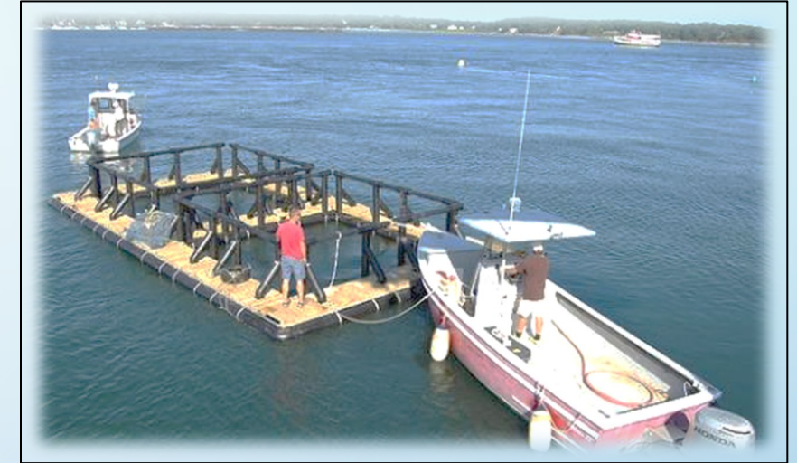
Deploy floating raft onto and 4-point mooring system
