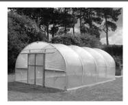
Our recommendation: Strong doors, strong structure. Poly cover buried in ground, frame anchored by anchor plates or burying. High resistance to high winds provided the door is secured.
