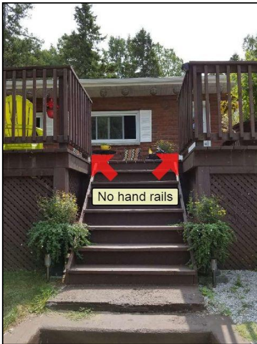
28. Poorly built
