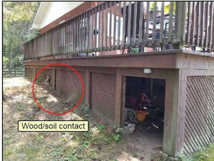
34. Poorly built
