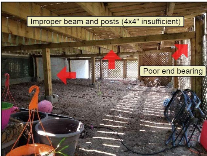
32. Poorly built
