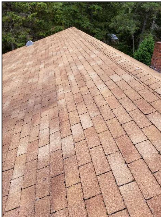
1. Asphalt shingles
