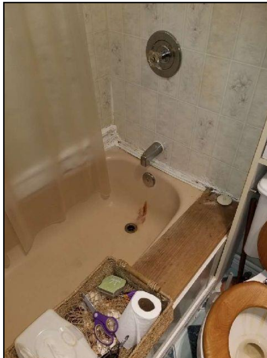
116. Not smooth, impervious or water resistant
