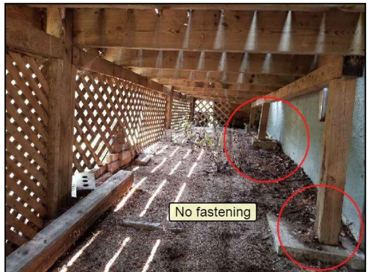
33. Poorly built
