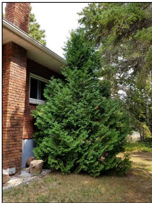
61. Large trees close to building
