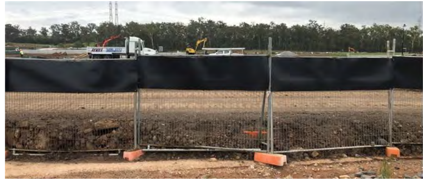
Inset 3: Indicative temporary fauna exclusion fencing aligning a construction site
