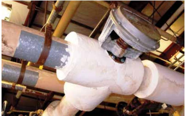
**In one installation, a three-way valve resulted in return water  $\Delta T$  of 60°F-80°F, and the rapid expansion and contraction damaged the boiler.**
