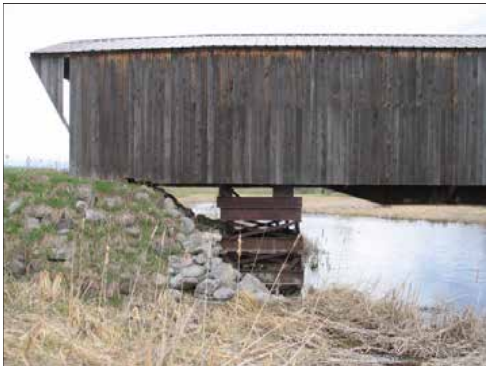
Figure 34. Covered bridge. View to the north (5/10/22).
