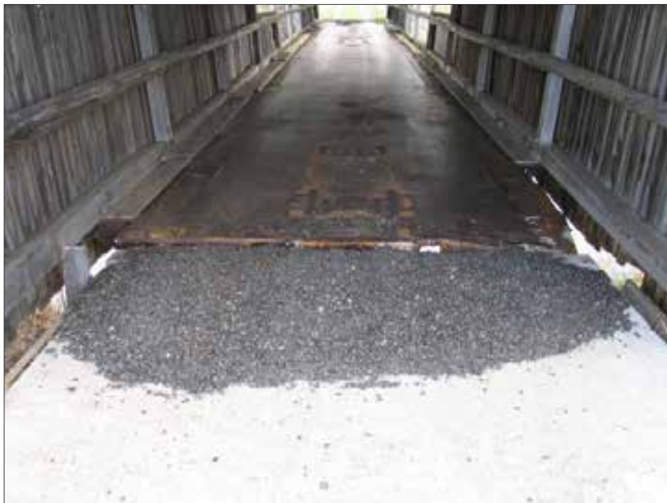
Figure 38. Covered bridge. Interior floor (5/10/22).
