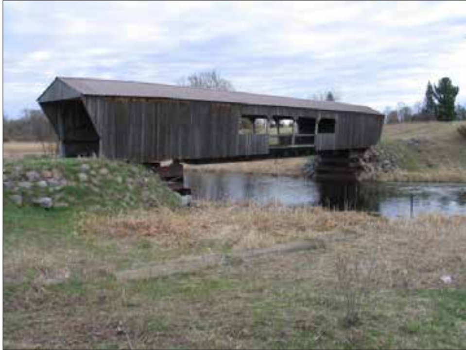
Figure 33. Covered bridge. View to the northeast (5/10/22).
