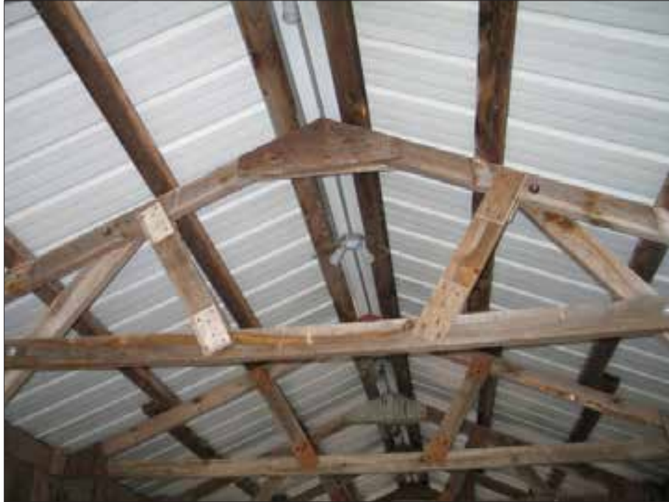
Figure 37. Covered bridge. Interior roof (5/10/22).
