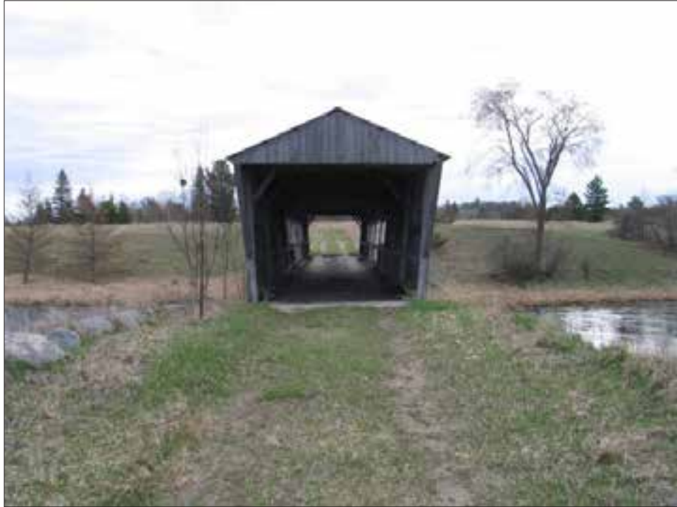
Figure 35. Covered bridge. View east-northeast (5/10/22).
