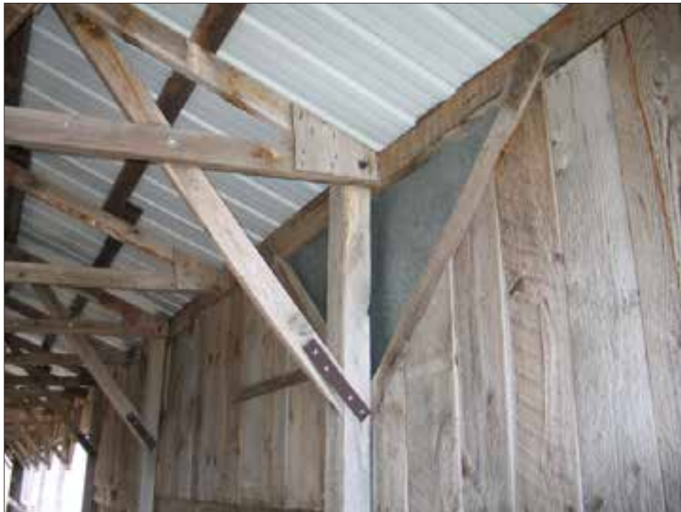
Figure 36. Covered bridge. Interior wall (5/10/22).
