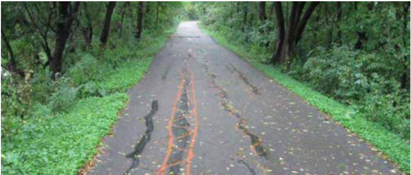
Cracks on the Gateway State Trail
