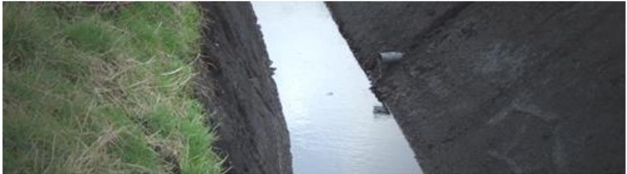
TG Drains has 2 purpose built buckets for the 12 tonne excavator that can dig a spoon drain or a "V" shaped drain. The excavator is laser guided ensuring an even grade in the drain.
