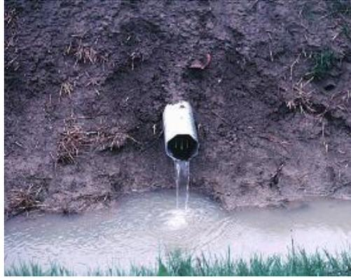
**Polydrain outlet to a drainage ditch**
