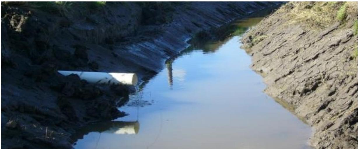
When the water table in the soil is higher than the polydrains, water flows into the holes of the corrugated polydrain. This lowers the water table to the depth of the drains over the course of several days. Subsurface drains allow excess water to leave the field, but once the water table has been lowered to the elevation of the drains, no more water flows through the drains.
