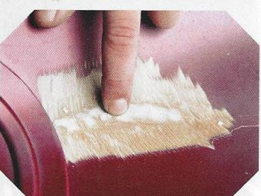
**24** Allow the mixture to dry, checking by touch after 15 minutes or so.
