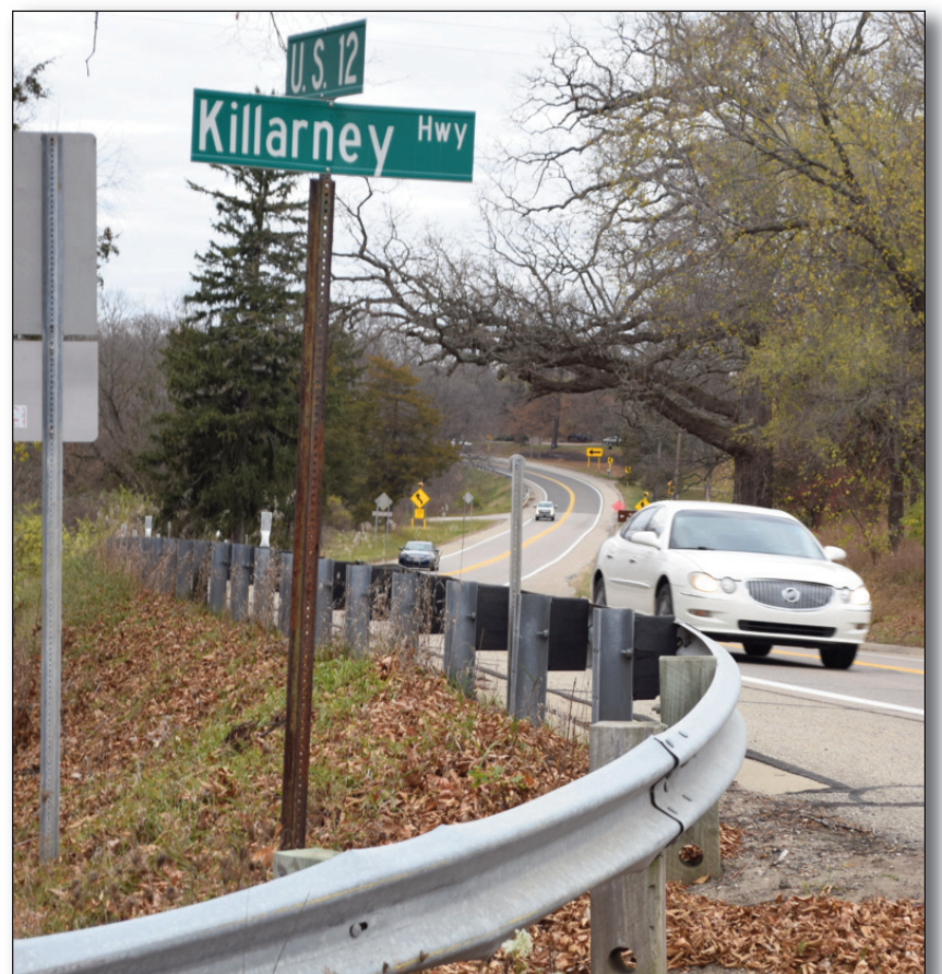
Above is the intersection of U.S. 12 looking northwest from Killarney Road. Trucks hauling product onto U.S. 12 would have limited sight distance when accessing the highway, particularly from the east.
