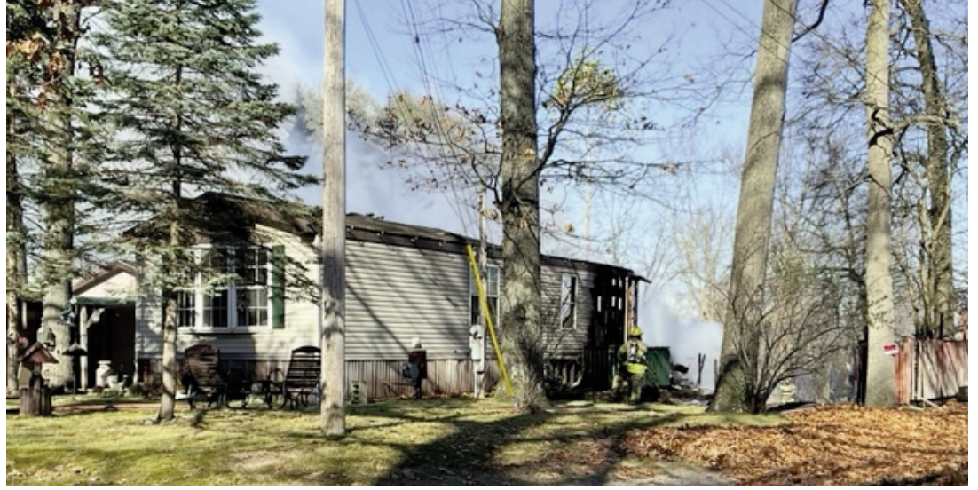
Fire destroyed a trailer in the 6000 block of Amberton Drive in Napoleon last Wednesday. The lone occupant residing in the trailer and a cat both made it out alive. COURTESY PHOTO
