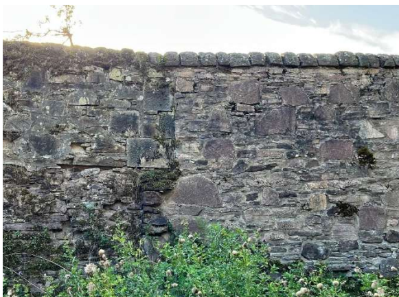
Photographs showing (left) – apparent infill to existing wall, note change in stone and coping types, and (right) – location of previous toilet block in area of wall to be removed
