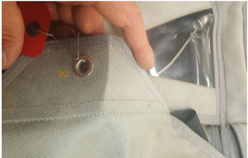
Figure 6. Plastic Stiffener Supporting the Grommet
