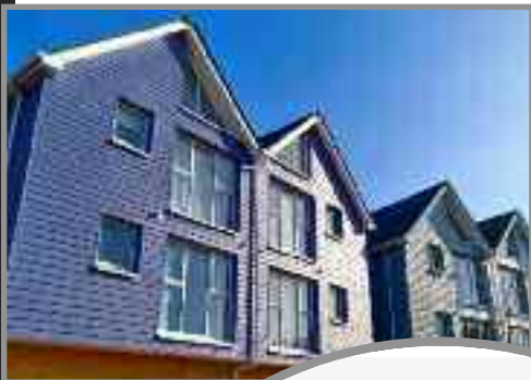
Fibre Cement Cladding.
