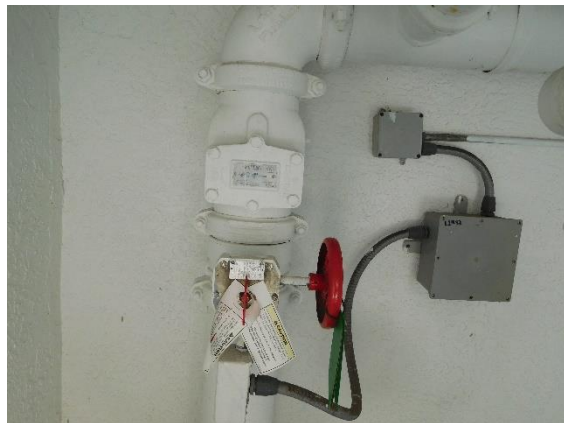
TYPICAL FIRE SPRINKLER CONTROLS
