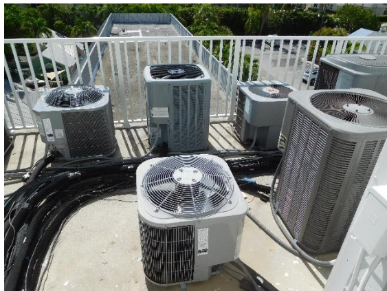
TYPICAL AIR-CONDITIONER UNITS
