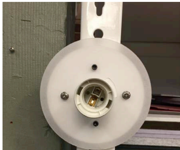
Base electrical plate mounted in place, according to template locations.
