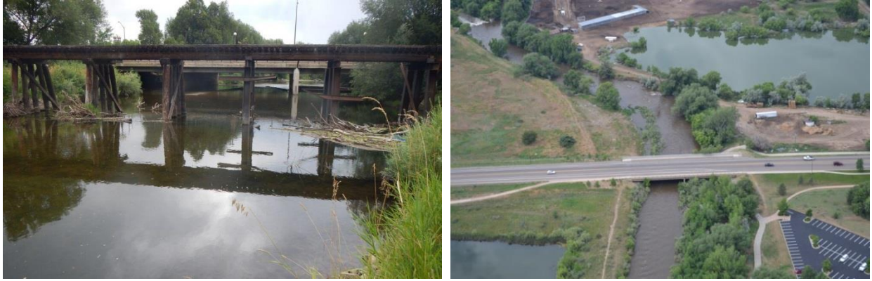
Figure 3.9: Twenty-two bridges span the Poudre in the study area. At left, a railroad trestle and College Avenue and at right Prospect Road.
