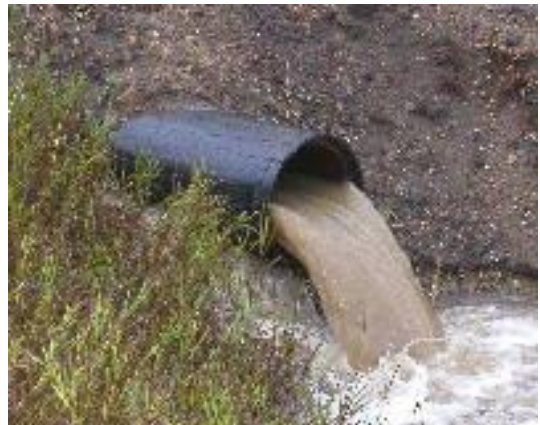
Figure 5.7: In addition to its construction site sediment and erosion control program, the City's LID Program requires on-site infiltration of stormwater to help prevent in-stream impacts associated with increased imperviousness.
