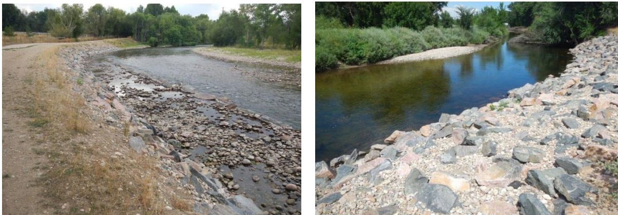
Figure 3.11: Bank and channel armoring is employed to increase channel resistance, protect above and below ground infrastructure or prevent river migration.
