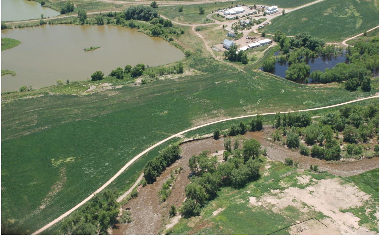
Figure 3.6 While open space and parks management of lands in the floodplain primarily has a positive influence of river health, infrastructure such as the bike bath in this photo is often located so close to the river that it's protection disconnects the river from a functional riparian zone .
