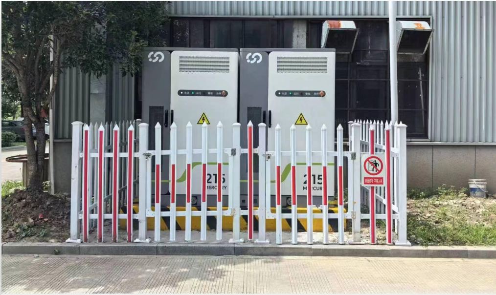
Project: Plastic Products factory size :200kW/430kWh location:Jiaxin city zhejiang province
