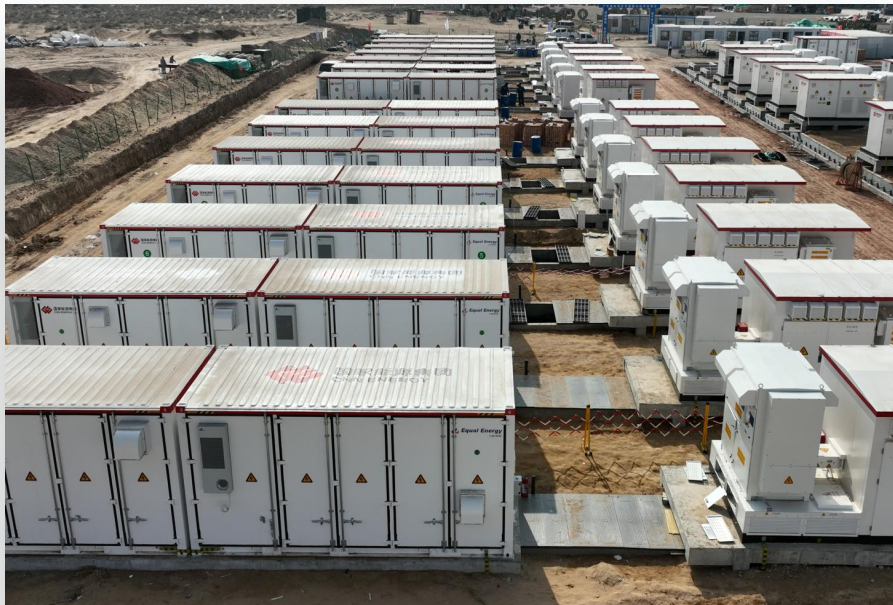
Project1.Independent energy storage plant 60MW/120MWh
