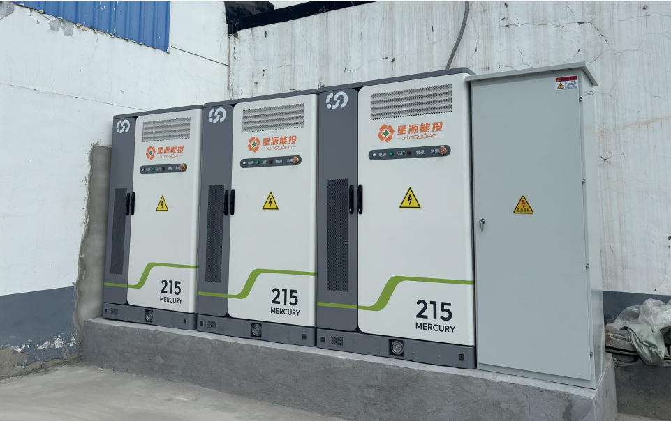
Project: Aluminum Material factory size :300kW/645kWh location:Suqian city Jiangsu province
