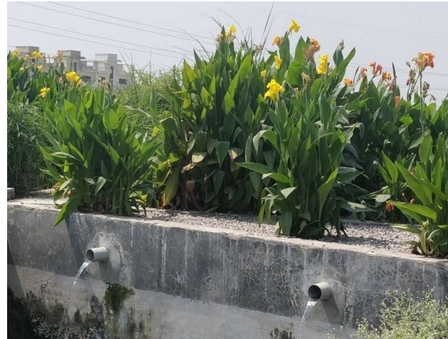
NRI CITY, KANPUR, (100 KLD)
