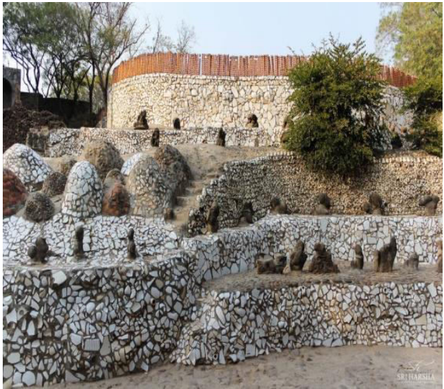
Glimpse of employing construction waste ( ref. from Rock Garden Chandigarh.
