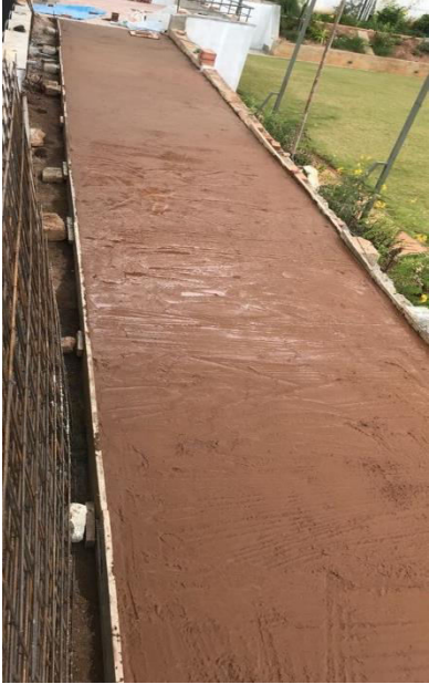
Mud Concrete Pathways
