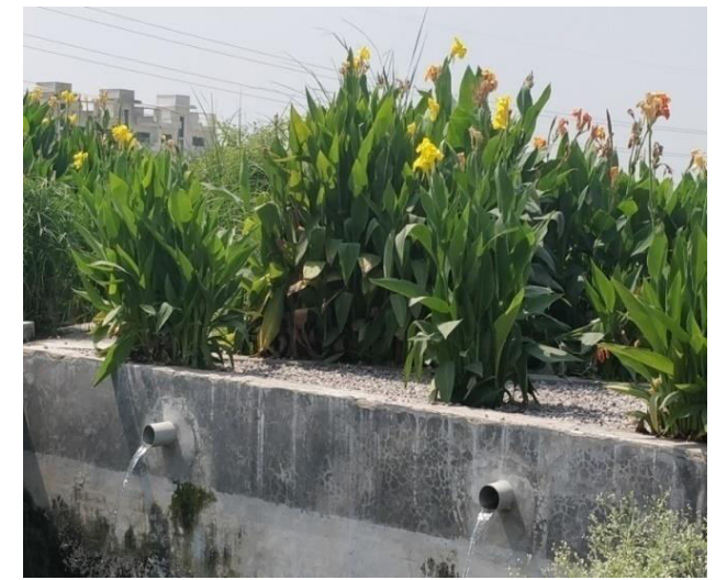
NRI CITY, KANPUR, (100 KLD
