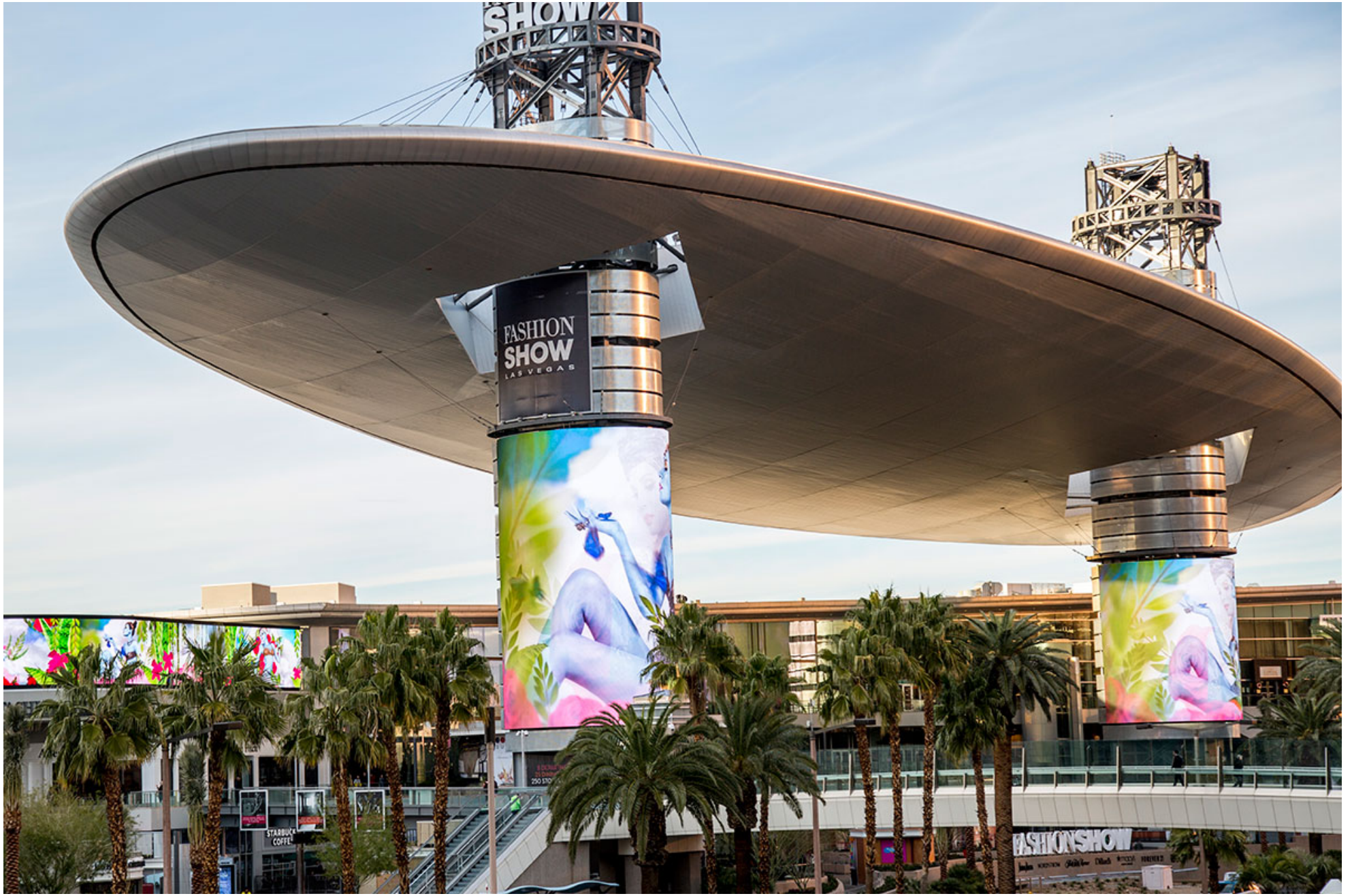
Systems in photo: Column Wrap
