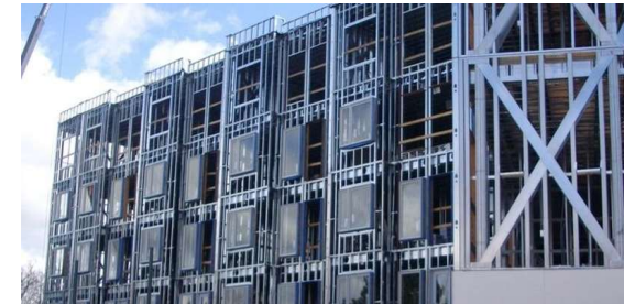
Multi-Storey CFS Construction
