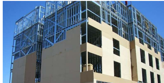
Mid-Rise / Mixed-Use Steel Framing
