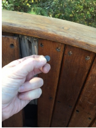
Figure 5: Plastic bungs made future beadboard removal easy
