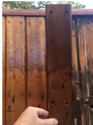
Figure 2: Cockpit beadboards were carefully removed to gain access to the hose
