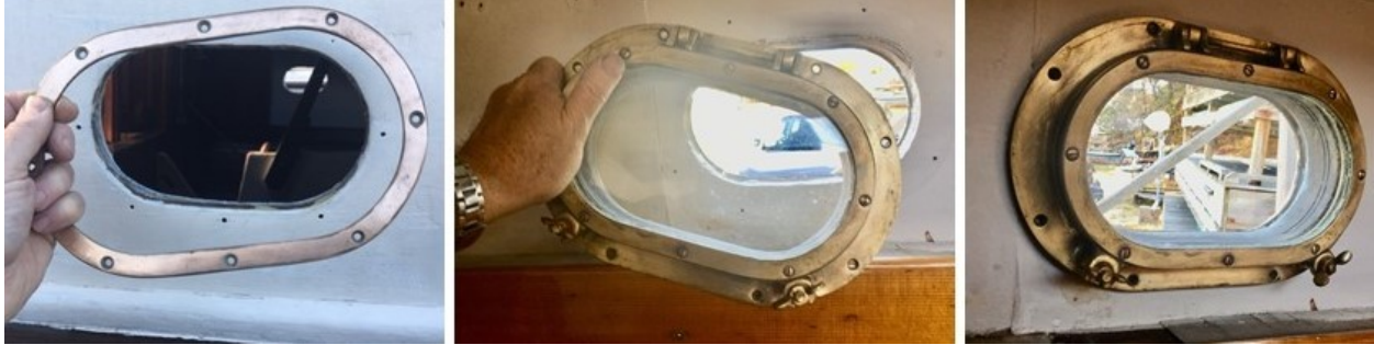
Figure 10: Porthole exterior surrounds and internal portlights were reinstalled
