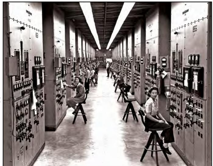
Women workers stationed at the control panels of the massive calutrons, a type of mass spectrometer developed during the Manhattan project for the purpose of extracting the Highly fissile isotope U-235 from nonfissile uranium. U-235 comprises less than 1% of uranium found in its natural state, and must be separated to a high level of enrichment to be useful for both nuclear power and nuclear weaponry. These ladies seen above were quickly known as "Calutron Girls".
