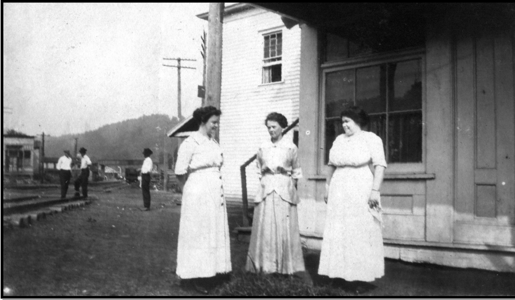
Delia Cross at left, standing with her sisters who were Wrights but not sure which is which. This picture would have been taken around 1908. The Cow Creek Trestle was built in 1904, and as you can see, it is in background. Delia was the wife of Luther Cross, and worked as a mail clerk in the Post Office. She died around 1920 at only 40 years of age. I believe this building is Keebler's Store, on the east end which also housed the Post Office until the new Post Office was built on Estabrook Avenue around 1910-12.
