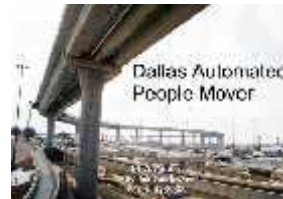
Dallas Ft Worth Airport Automated People Mover
