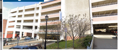
Scovill Street Garage
