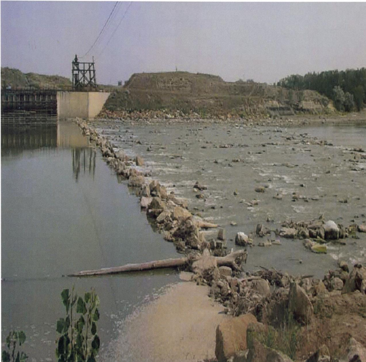
Intake, Montana water intake diversion structure on the Yellowstone River
