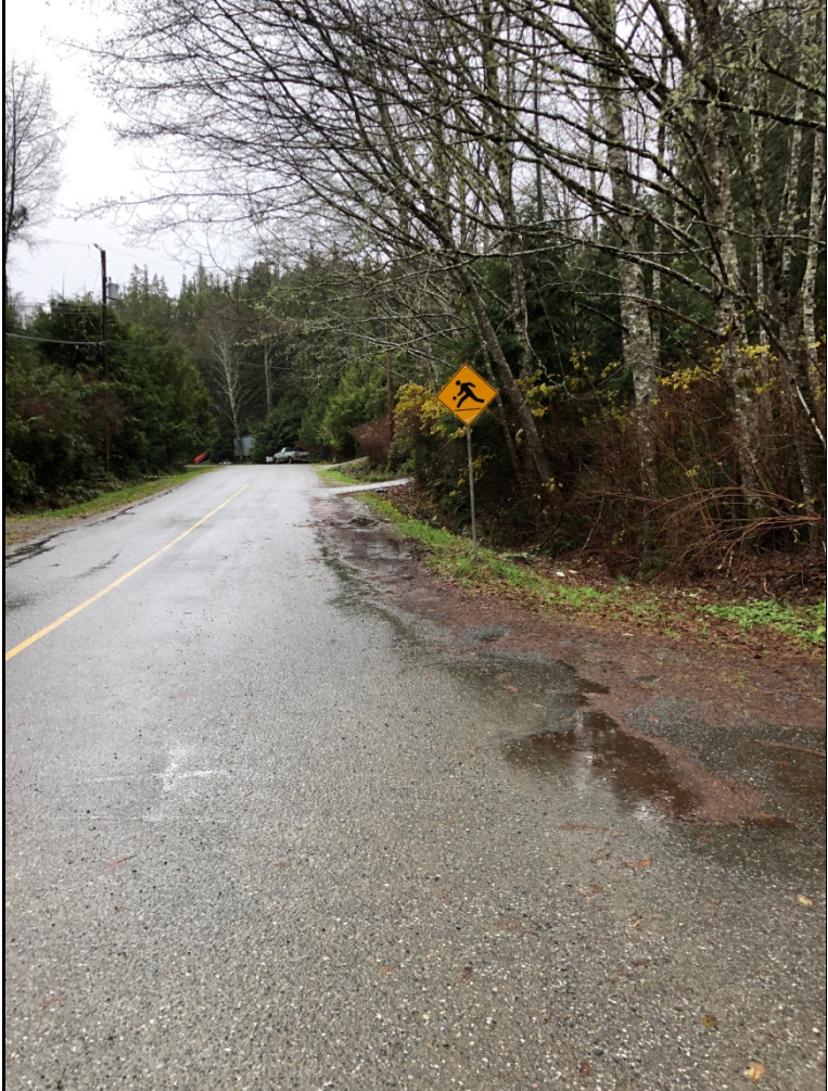
Appendix A.4 - Leighton Way (facing southwest)
