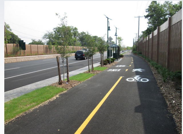
Photo of completed section of NY 347 in Hauppauge/Smithtown. NYS DOT had developed this Complete Streets concept for the entire length of NY 347, from Hauppauge to Mt. Sinai in the Towns of Smithtown and Brookhaven. The noise walls are constructed in residential areas that abut NY 347. Improvements include a shared-use path along the south side of the roadway and bus stop shelters.
