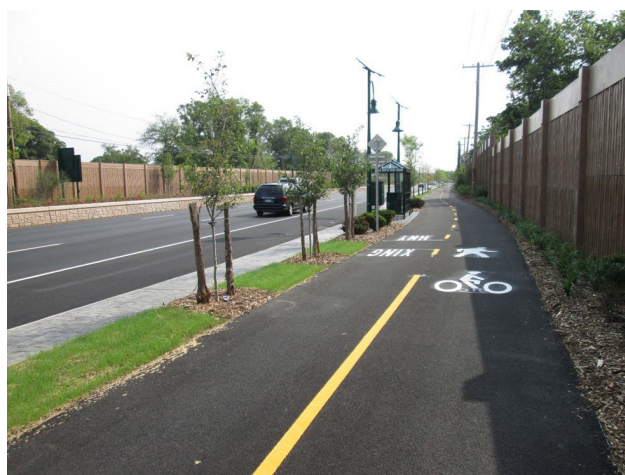
Photo of completed section of NY 347 in Hauppauge/Smithtown. NYSDOT had developed this Complete Streets concept for the entire length of NY 347, from Hauppauge to Mt. Sinai in the Towns of Smithtown and Brookhaven. The noise walls are constructed in residential areas that abut NY 347. Improvements include a shared-use path along the south side of the roadway and bus stop shelters. Source: Google Earth
