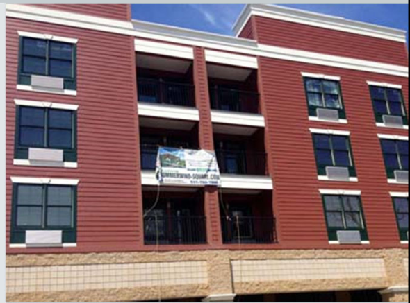
Summerwind Square on Peconic Avenue Source: Riverhead News Review – Times Review
